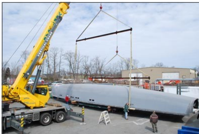
Goetz Safely Rolls an 82' Composite Part
